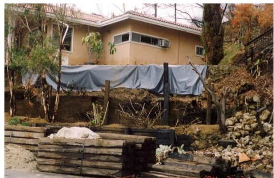
20415 Little Rock Way. Replacing burned railroad ties with highly flammable railroad ties.
