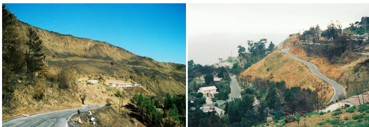
Barley contouring slopes before covering them with straw. Germinated barley in contours along Big Rock Dr.
