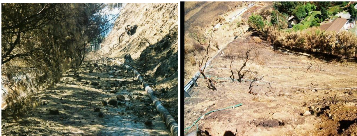
Old Seaboard-Big Rock Connector Rd. with water main. Temporary irrigation lines above scorched pine
