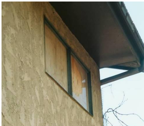
Post fire: Broken window at fire-catcher overhang. Melted pipes, fire-stopped vent cover.
