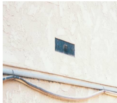
Post fire: Broken window at fire-catcher overhang. Melted pipes, fire-stopped vent cover.
