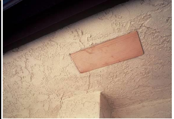
Preparing for a wildfire by protecting windows and vents on a stucco home.
