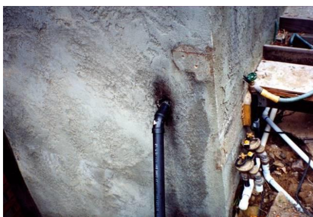
Fire entry through stucco siding of burned pipe (replaced)
