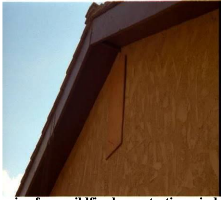
Preparing for a wildfire by protecting windows and vents on a stucco home.
