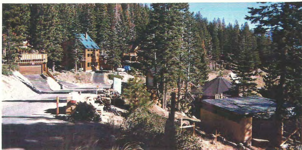
Photo 12. New homes along lower Tyner Drive in Incline Village are characterized by fire-safe roofing, reflecting a change in the fire-safe building codes. Since the wood shingle roof is the greatest single factor in structural losses during wildfires (and often in spreading the fire to adjacent homes), a fire-safe roof will eliminate the greatest fire threat to a home. While a home with a wood shingle roof rarely survives a wildland fire unattended, a home with a fire-safe roof, depending on distance and amount of clearance of flammable vegetation, increases its odds of surviving a wildland fire unattended under the same conditions by at least 20 times, or 2000%. These are the best odds offered to any gambler anywhere in Nevada. The odds are further increased in favor of homes with fire-safe roofing as wildland fire protection agencies are being trained to protect homes that have a chance of surviving a wildfire with minimal tie-up of equipment and labor and bypass homes whose chances are minimal. Thus when a wood shingle roof catches on fire in a wildland fire conflagration, it is normally a total loss (R.#39-31; 11-11-89).
