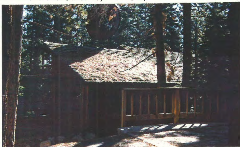
Photo 8. Pine needles from adjacent dying trees are covering the wood shingle roof of this house along Valley Drive in Incline Village. Such apparent disconcert or lack of awareness of the extreme fire danger often results through absentee ownership. It must be reemphasized that one is often only as safe as his neighbor. A neighbor (private homeowner as well as public agency) thus has a legal responsibility not to endanger the life and property of surrounding homeowners (R.#39-29; 11-11-89).
