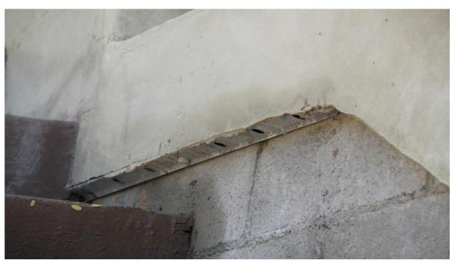
This weep screen is located adjacent to the concrete entrance staircase and just above a proposed small planter, still an Achilles heel in a fire-safe designed home.
