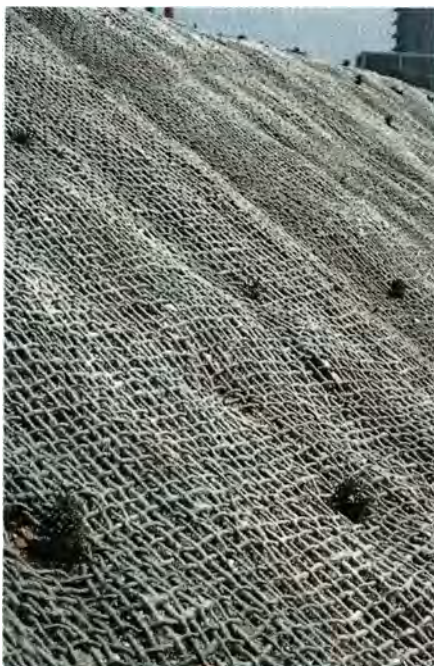
Erosion netting reduces soil erosion on steep slopes.
