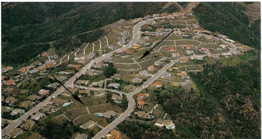
Bench drains (arrow) enhance slope stability; they break up the length of the slope and allow a greater choice of species for landscaping.
