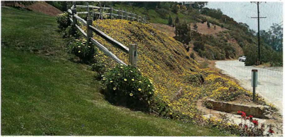
This sloping lawn sheds water onto the adjoining bank, causing slippage.
