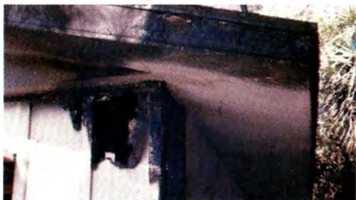
Boxed eaves that prevent heat entrapment even if the wood siding catches on fire.
