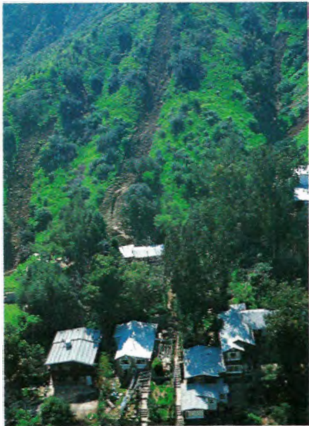
Slope failures after annual grasses have replaced the deep-rooted native vegetation.
