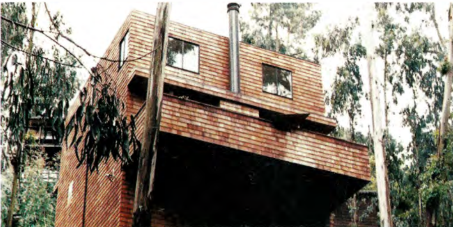
Wood sidings are almost as fire-prone as wood roofs.
