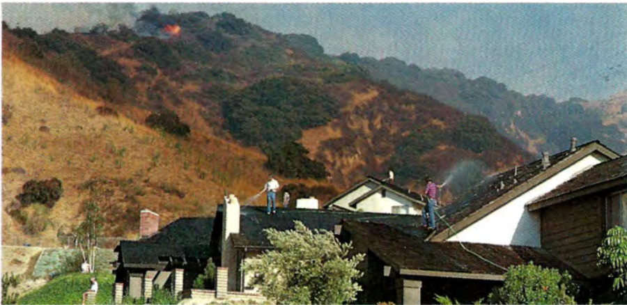
Wood shingle roofs require an inappropriate amount of manpower and water during a wildfire because they are easily ignited by flying sparks.
