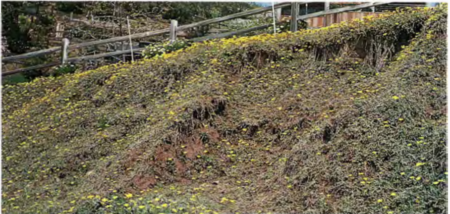
Capeweed on the bank is excellent to prevent surface erosion but its shallow root system is unable to prevent soil slippage.
