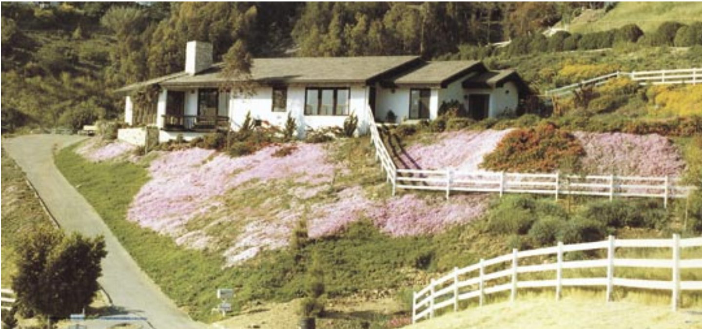
This home, designed to be fire-safe, also has a 30-foot setback safety zone.
