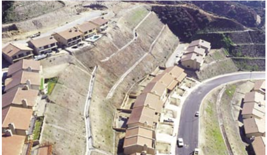
Planting the right plant in the right place is as important on manufactured slopes (foreground) as on natural slopes (right background).
