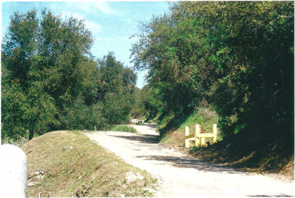
Photo 12 – An additional concern are the narrow, winding roads with inadequate clearance. Such roads are not safe to pass during the burnout period of the surrounding flammable vegetation despite the presence of an occasional fire hydrant that may give a sense of false security (4-5-2000)
