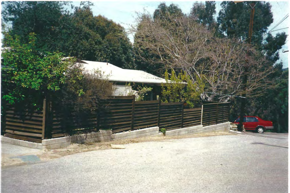
Photo 9 – Wooden fences are also a fire fuse and transmit not only the heat but the flames of the fire directly onto the home and unprotected windows (Roll #43-22, 3-25-2000).
