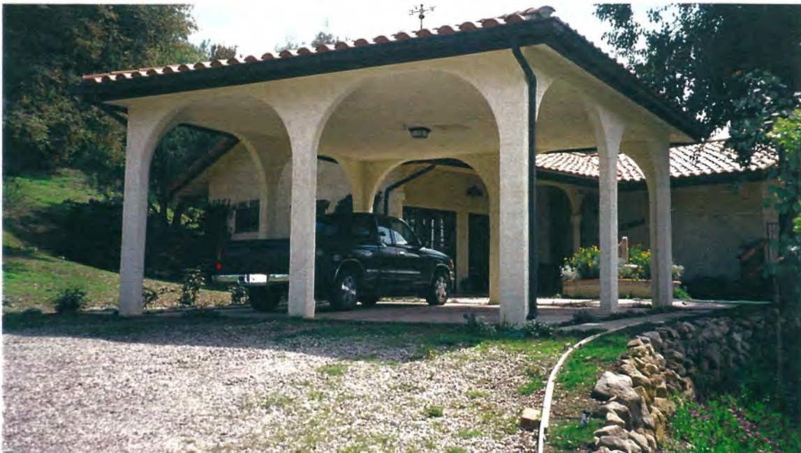
Photo 3 – The Hillsteads rebuilt their carport as probably the most fire-safe carport in Topanga! It has a fire-stopped red tile roof, with stucco siding, an adequate firebreak, and no attached wooden structures (Roll #34-3 3-25-2000).
