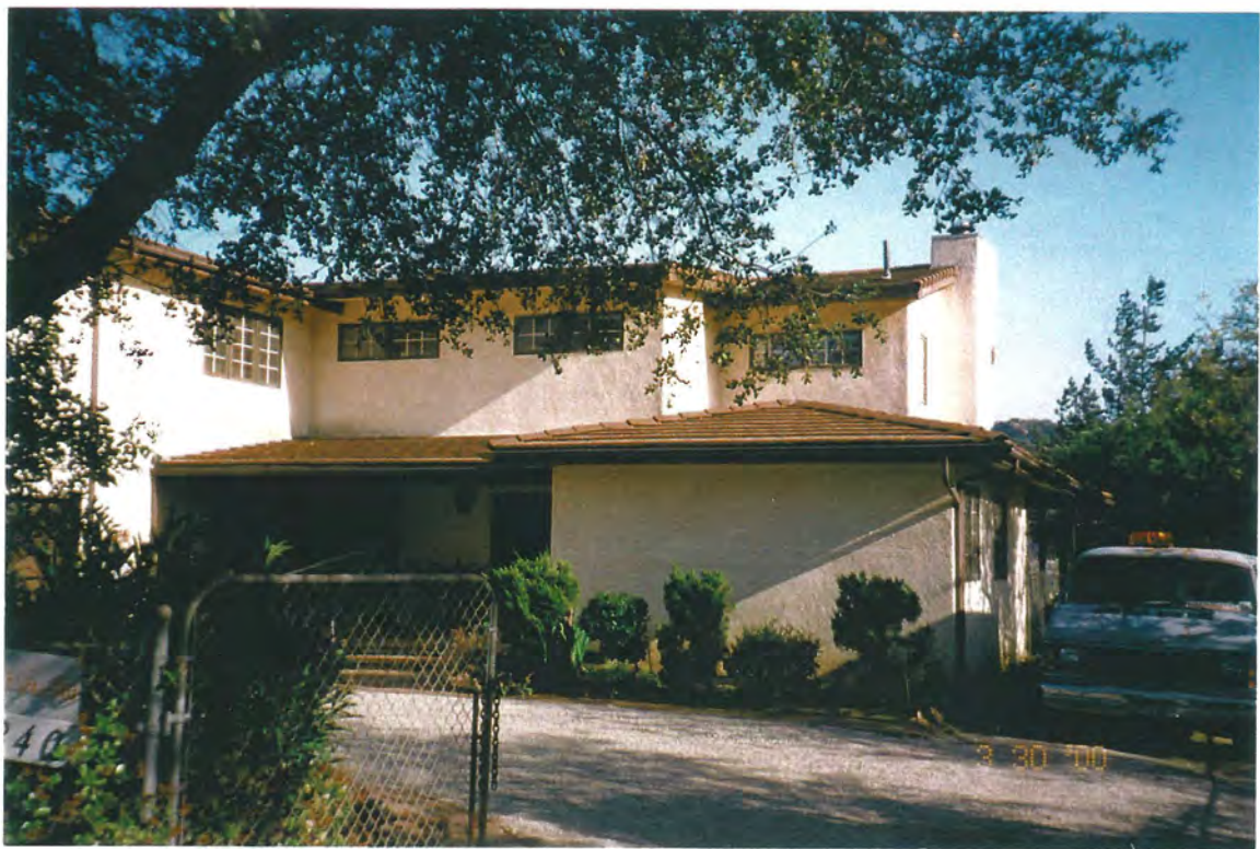
Photo 4 – The Mosses also rebuilt their home as a basically fire-safe designed structure with a tile roof, stucco siding and dual-glazed windows, with flammable fuels, inclusive of landscape fuels, removed from the windows and also largely from around the house (Roll #365-10 3-31-2000).
