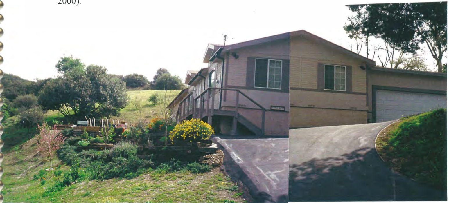
Photo 5 – The former Morgan home on Callon Drive was rebuilt as a double trailer with attached garage and generally adequate clearance. However, it still sits at the top of a minor draw (separated by Callon Drive) vegetated largely with Bluegum Eucalyptus trees. The railroad tie planter boxes are also extremely difficult to extinguish once ignited and have the habit of re-igniting (just like some trick birthday candles) after they have apparently been extinguished. Pine trees along Callon Drive have also increased in size since the 1977 Fire (Roll #34-23/24; 3-25-2000).
