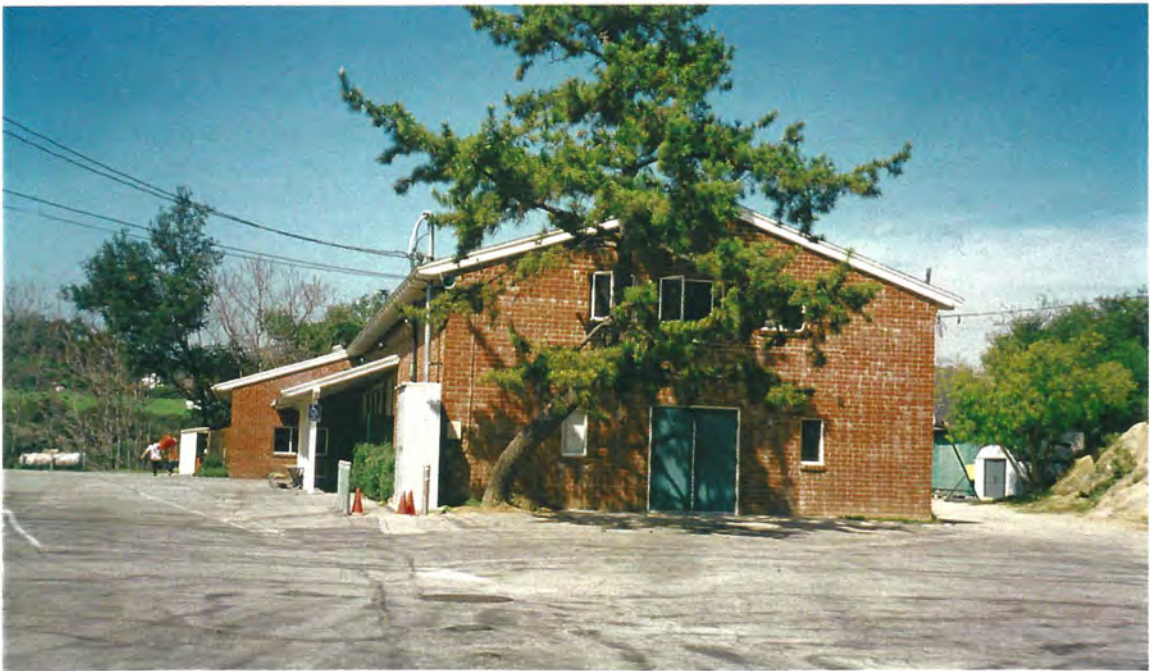
Photo 13 – Th old Topanga Community House, while basically fire-safe built, should also not be left unattended during a wildfire as surrounding structural storage fuels and the woody vegetation largely on its downhill northern slope could generate enough heat or firebrands that could break a window. The Community House can serve as an emergency fire-safe refuge shielding people trapped in the general area from the heat of the passing fire but can not serve as either a command post or evacuation center because of its size, its location in the midst of a fire area with only one access road and an exposed parking lot (not shown in this photo) (4-5-2000).
