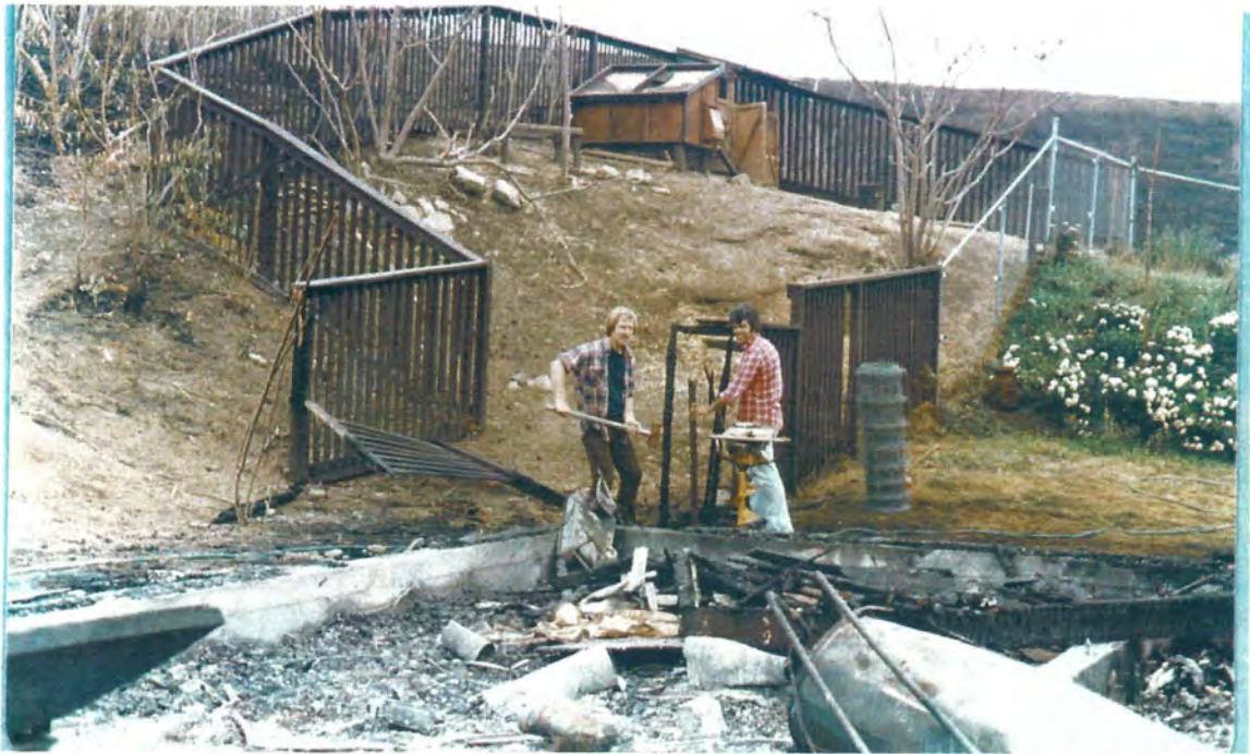
Photo 2 – The Hillstead home, a wooden house on Callon Drive, ignited (or re-ignited) hours after the fire had passed. As shown here in the 1977 photo from the photo album of Dick Hillstead, a relatively light intensity fire burned around the house and did not even catch the wooden fence of the livestock pen nor the wooden goat ‘house’ on fire. The goats and geese, huddled in the back of the pen, also escaped unharmed as the home burned down.
